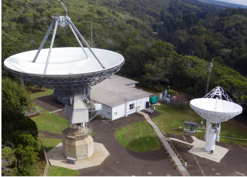
Figure 1: Two VLBI stations at Kokee Park, Hawaii: 20 m KOKEE and KOKEE12M that are 31 meters apart. The height difference of movable elevation axes is 8 meters.
